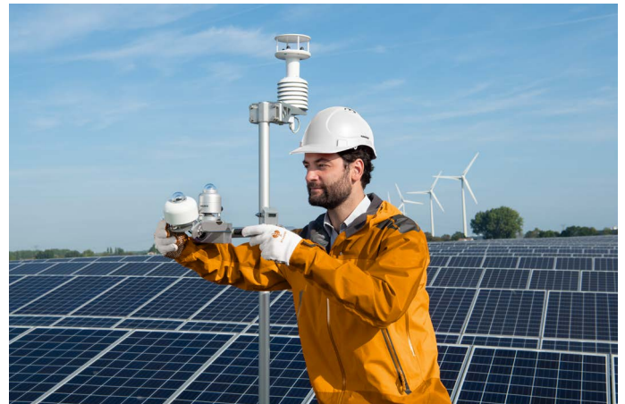
Figure 1 Two SR300 Class A pyranometers measuring GHI (Global Horizontal Irradiance) and POA (Plane of Array) in a PV performance monitoring system. How many of these systems should there be on a power plant?
