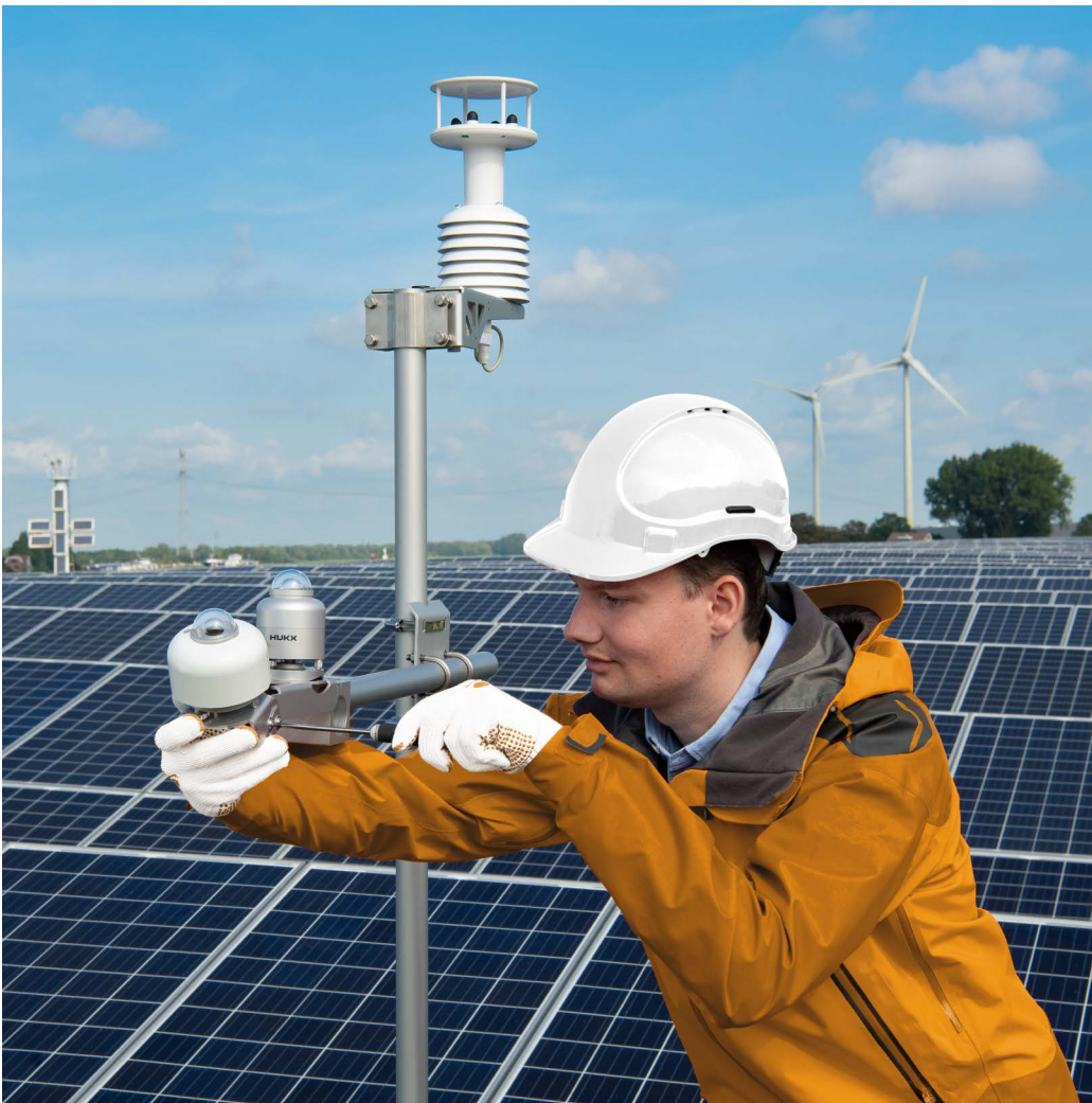
Figure 2 Typical use of pyranometers at PV power plants. The above picture shows two SR200-D1 pyranometers, one tilted for Plane of Array (POA) measurement (left), and another mounted horizontally for Global Horizontal Irradiance (GHI) measurement (right).
